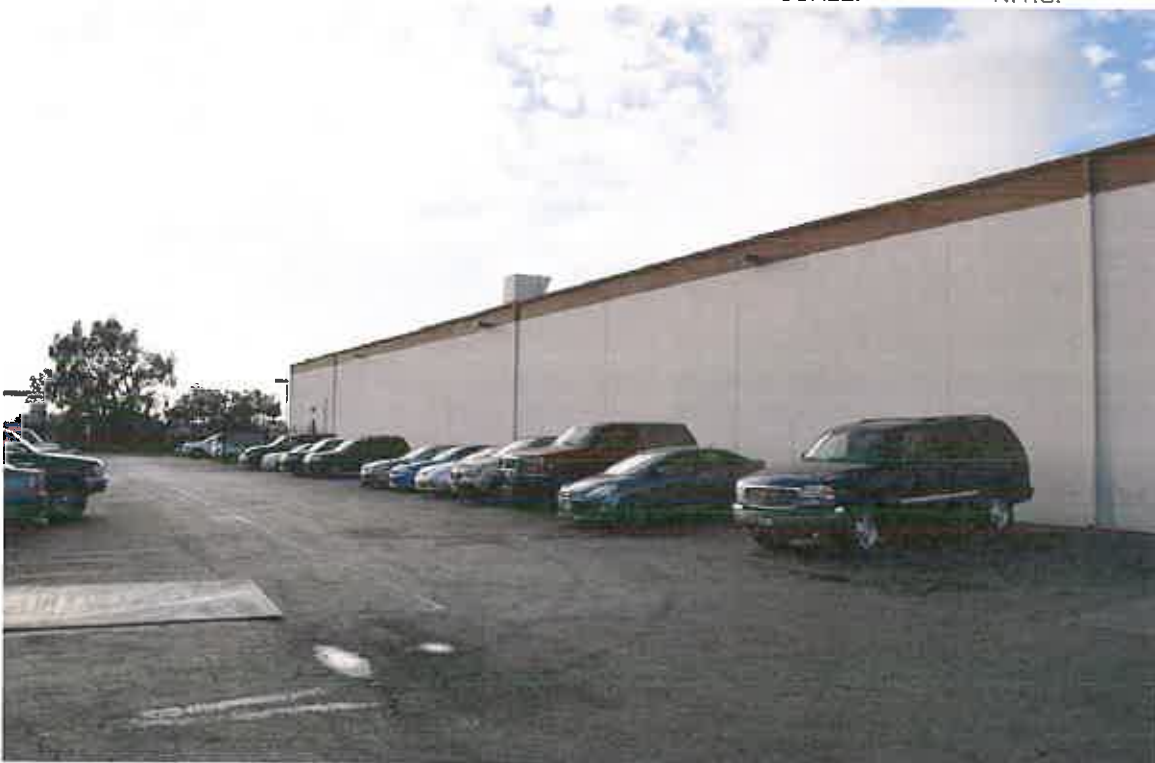
OVERALL SIDE PHOTO
