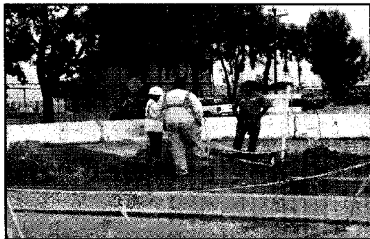
Street / Infrastructure Improvements
