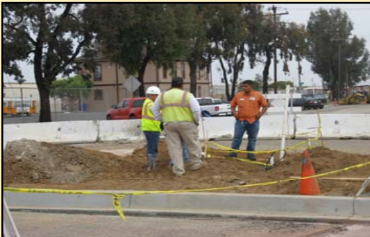
Street / Infrastructure Improvements
