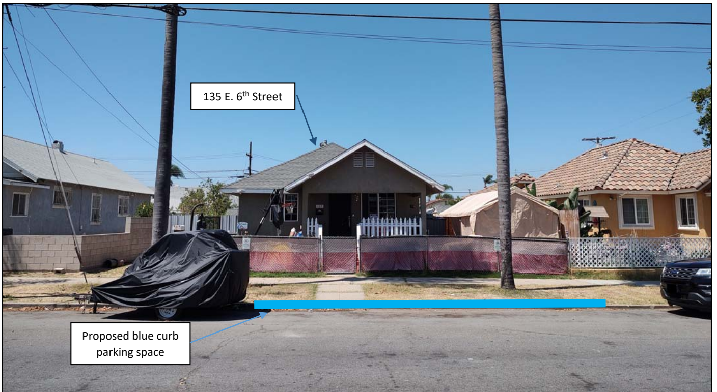
Location of proposed blue curb disabled persons parking space in front of 135 E. 6 th Street (Looking North)
