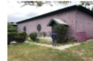
Current Accessible Entry
