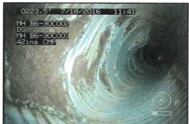
CORROSION IN PIPE WALL AND VOIDS TO BE GROUTED IN EXISTING 42" CMP
