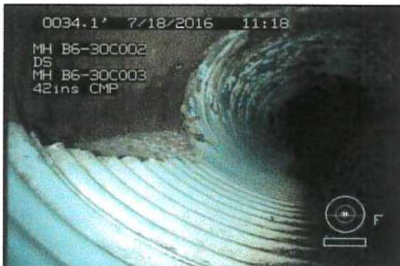
DEBRIS IN EXISTING 42" CMP STORM DRAIN
