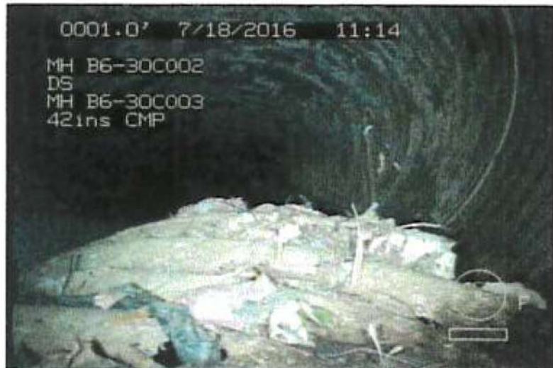
DEBRIS IN EXISTING 42" CMP STORM DRAIN
