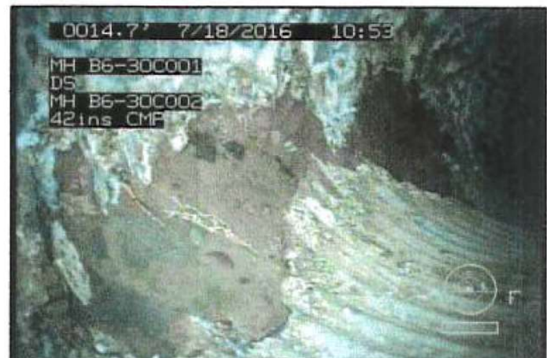
CORROSION IN PIPE WALL AND VOIDS TO BE GROUTED IN EXISTING 42" CMP
