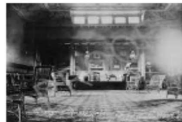
Interior Looking towards Mezzanine
