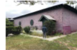
Current Accessible Entry
