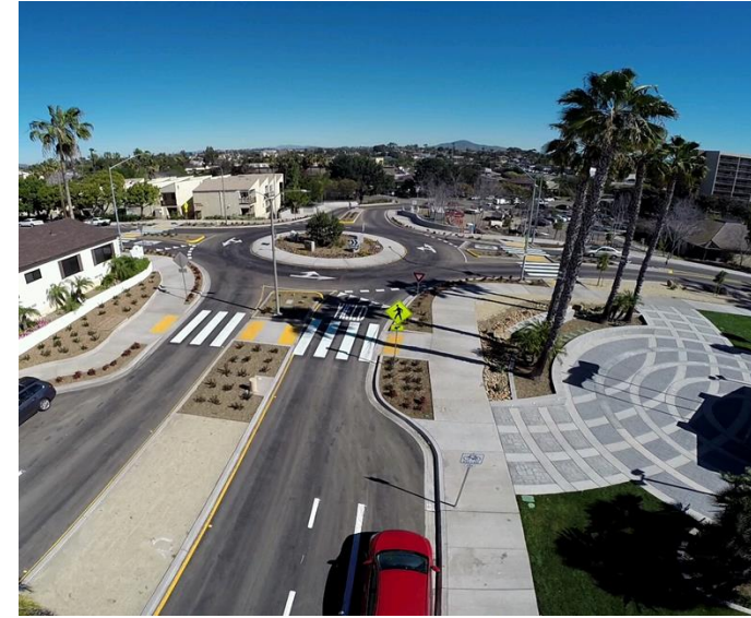
D Avenue & E. 12 th Street Roundabout Improvements
