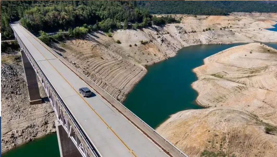
Bridge over Lake Oroville
