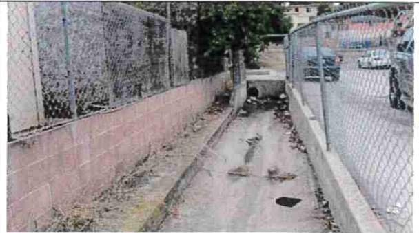
#8 – Looking southwesterly parallel with the alley.
