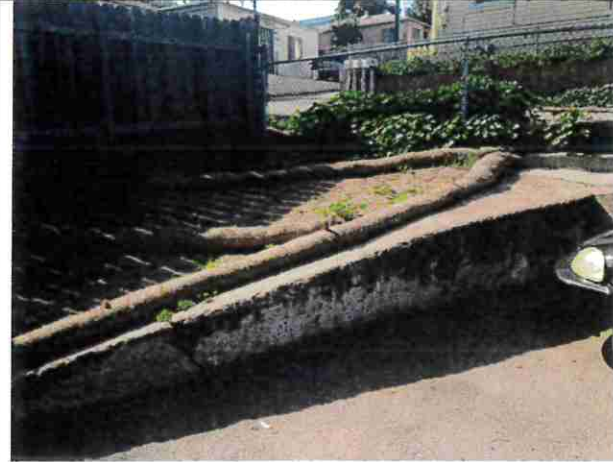
#13 – Looking southwesterly at the northeasterly corner of the site from the alley, with 'M' Ave. in the background.
