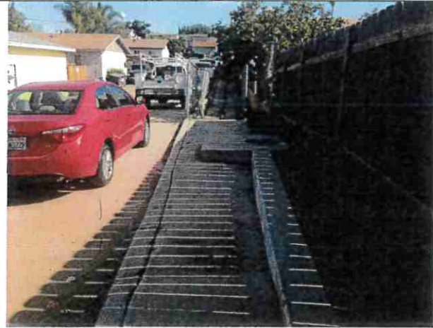
#9 – Looking northeasterly parallel with the alley.
