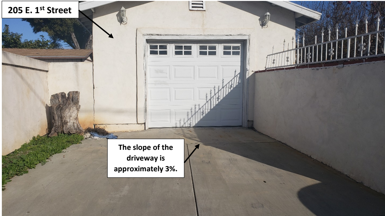
Existing driveway and garage for 205 E. 1 st Street (looking east)
