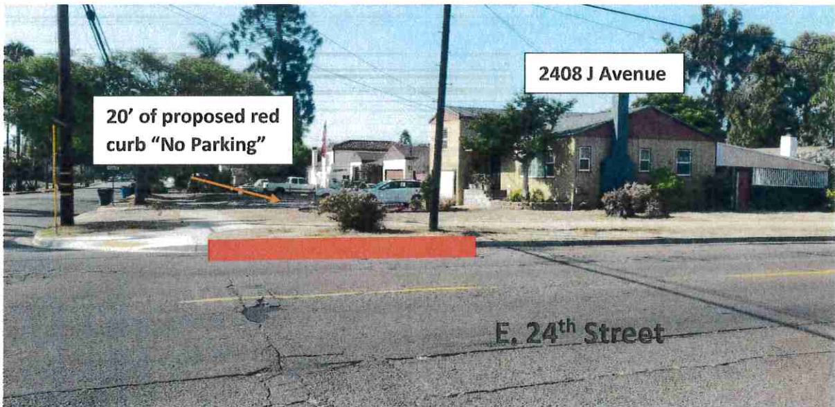
Location of proposed red curb "No Parking" on E. 24th Street (looking south)
