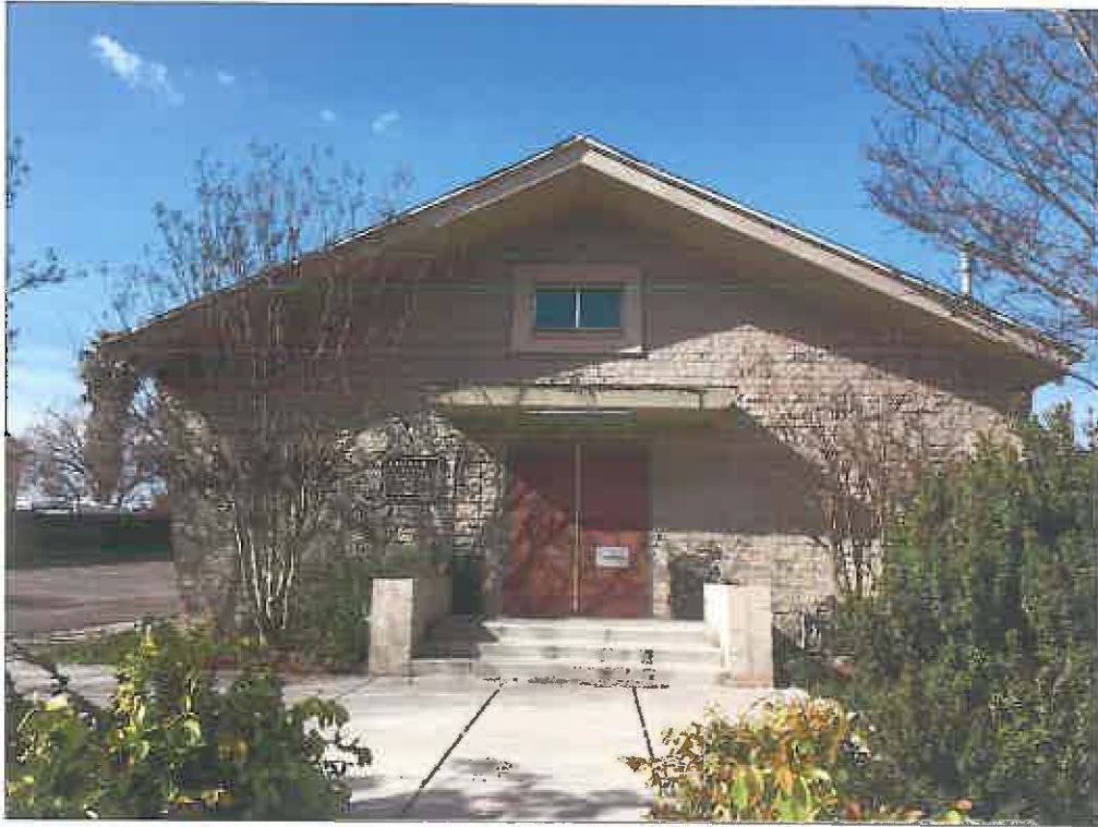
Front of building looking north from East 12 th Street
