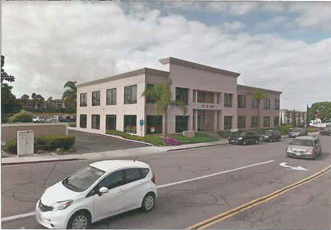
Existing building looking southwest from West 35 th Street
