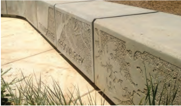
Concrete seat-wall with organic pattern
