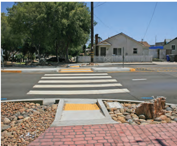
Curb extension and median refuge on Plaza Boulevard
