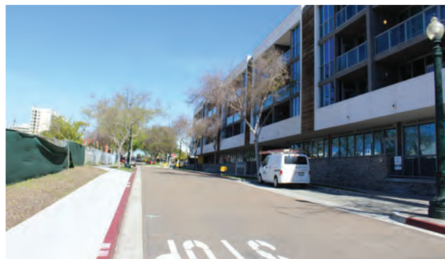
Existing green street
