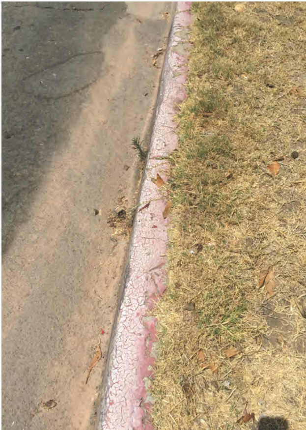
Figure 5-8: Inadequate Curb Marking Example
