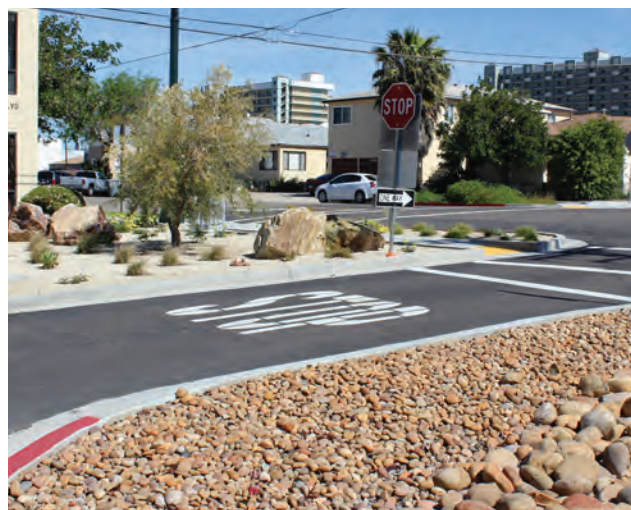
Curb extension and bioswale on Plaza Boulevard
