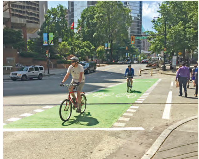
Intersection markings provide additional safety & comfort
