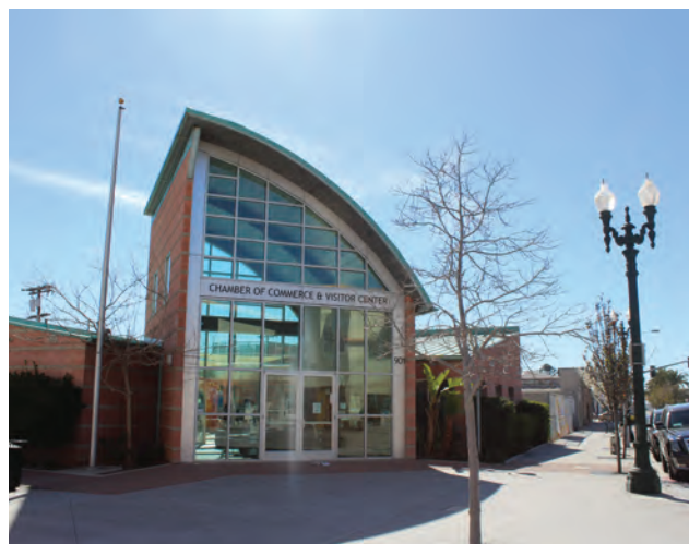
Chamber of Commerce glass façade uses clear non-reflective glass creating a desirable street-level building transparency
