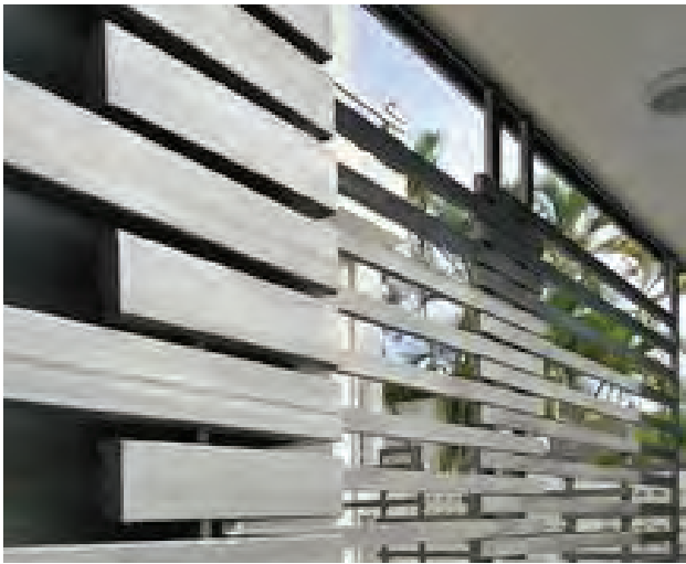
Concealing building facade treatment
