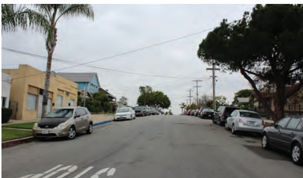
Existing residential street
