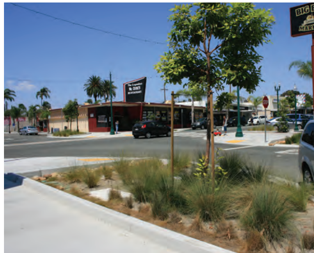
Storm-water bioretention areas along 8th Street
