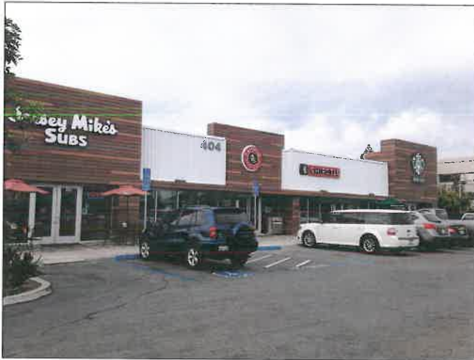
Existing building looking northwest
