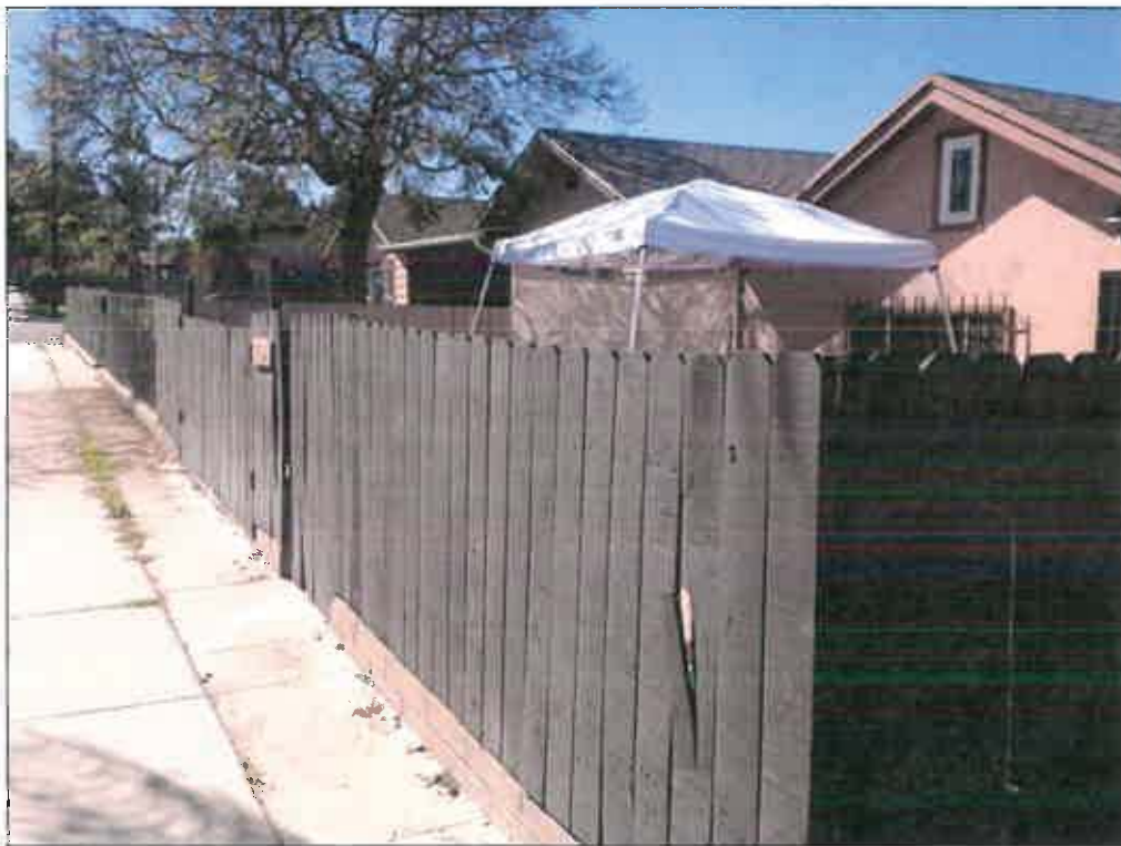
Fencing along east property line looking southwest
