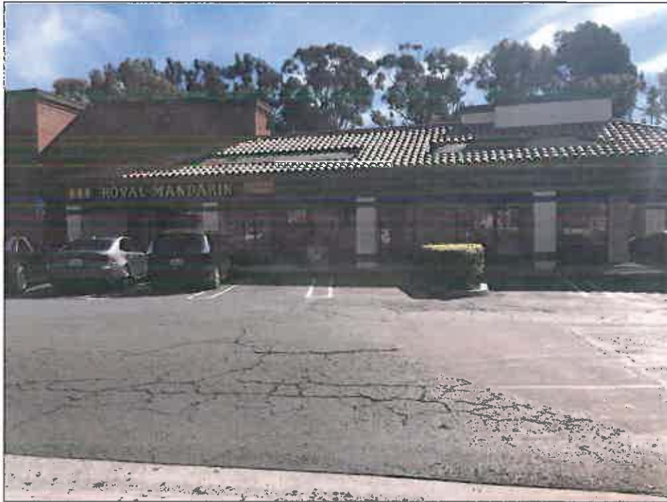
Existing restaurant looking south
