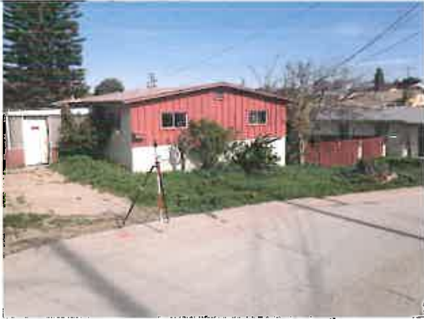
#1 – Looking northeasterly from 17 th St.
