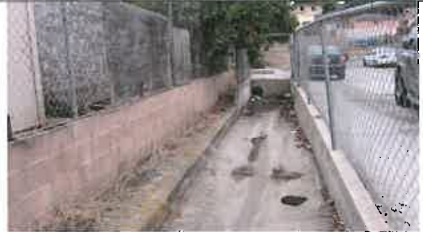
#8 – Looking southwesterly parallel with the alley.
