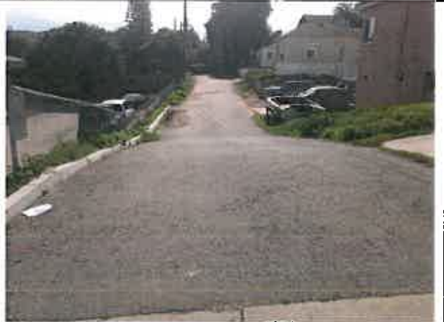
#12 – Looking southeasterly at 'M' Ave. from 16 th St.
