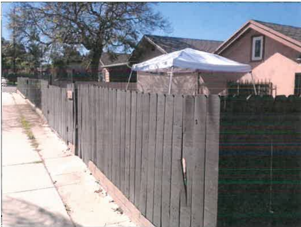
Fencing along east property line looking southwest
