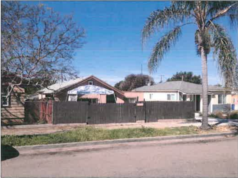
Front of existing house looking west
