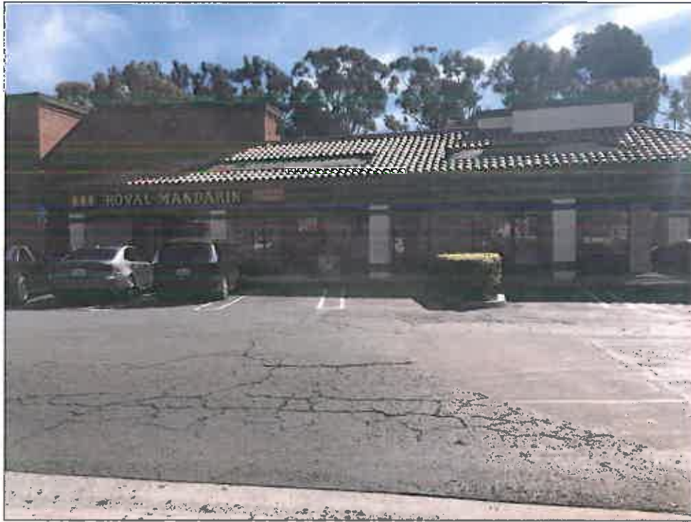
Existing restaurant looking south
