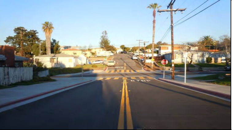
Safe Routes to School improvements approaching intersection of Palmer Street and Earle Drive near Palmer Way Elementary School (looking east)
