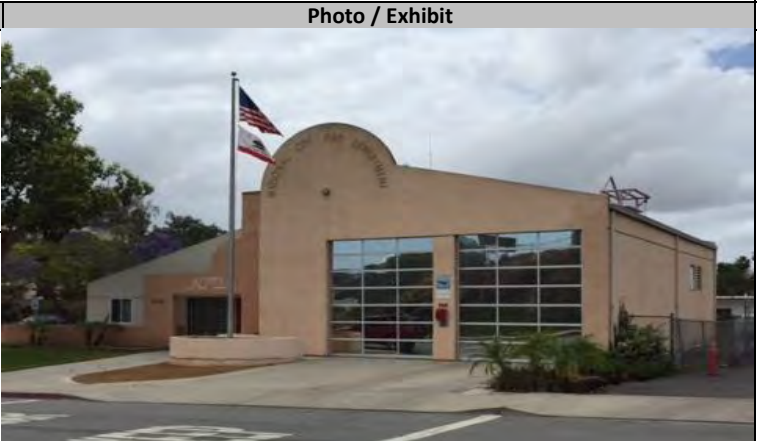
Fire Station 31 located at 2333 Euclid Avenue (looking northwest)
