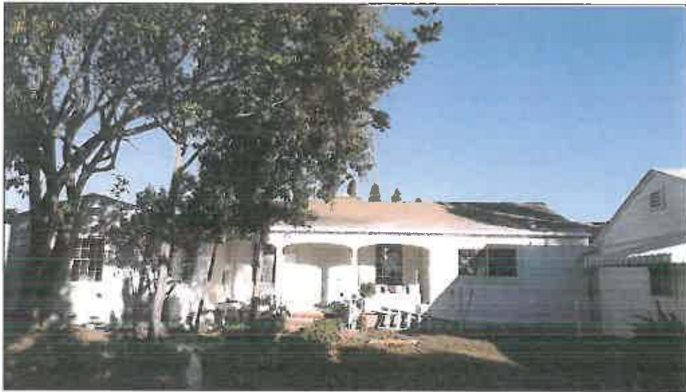
Existing home looking north
