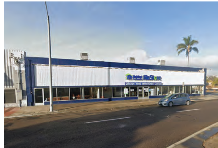
310 National City Blvd
