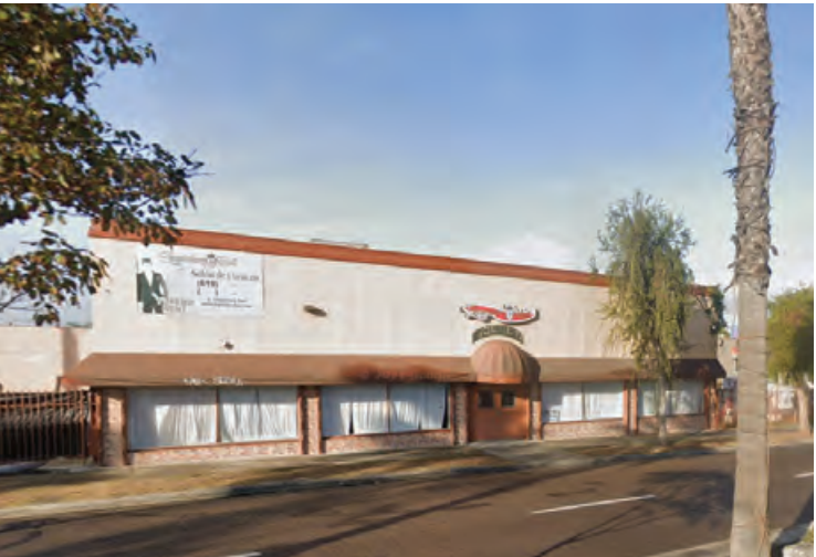
540 National City Blvd
