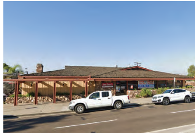
214 National City Blvd
